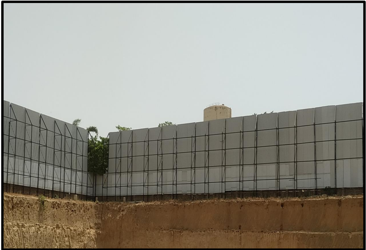
Inside - Rear Road Barricading
